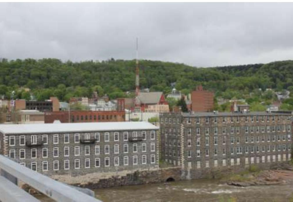
Former textile mills in Little Falls. Notice the arch for water return between the two mills.
