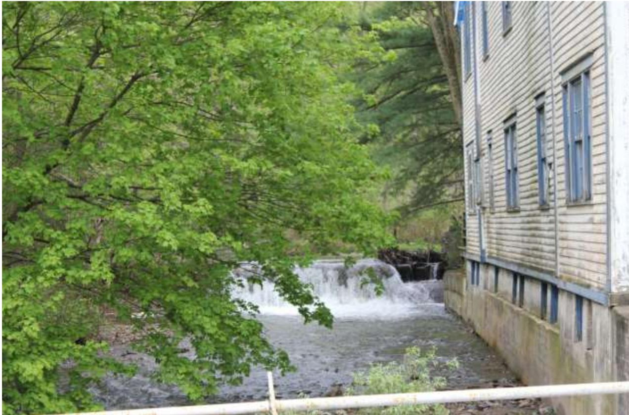
A former mill in Clayville. Notice the dam at left and the opening for the millrace between the whitewater of the dam and the mill building.
