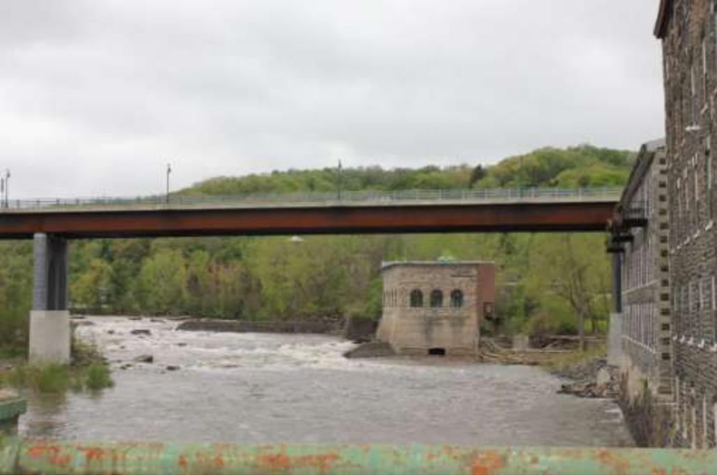
Mohawk River, Little Falls. Water was diverted using the dam in background of picture, turned turbines in the mills at left, and then exited back into the river.
